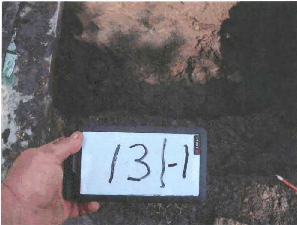
Picture 2: UST 131Banyan-1 tank pit after removal of tank.
